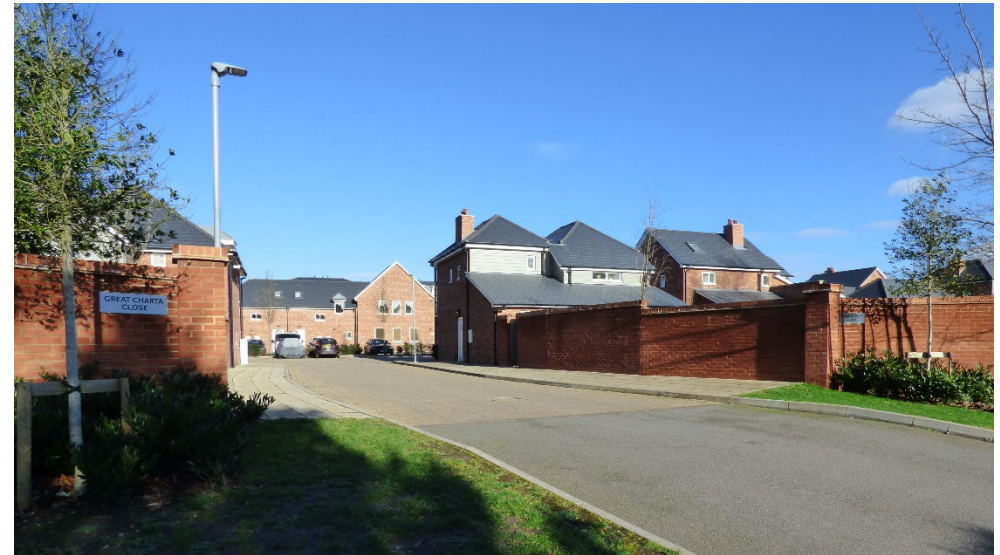
Figure 56: The high density of development of Great Charta Close urbanises the setting of the Conservation Area.
