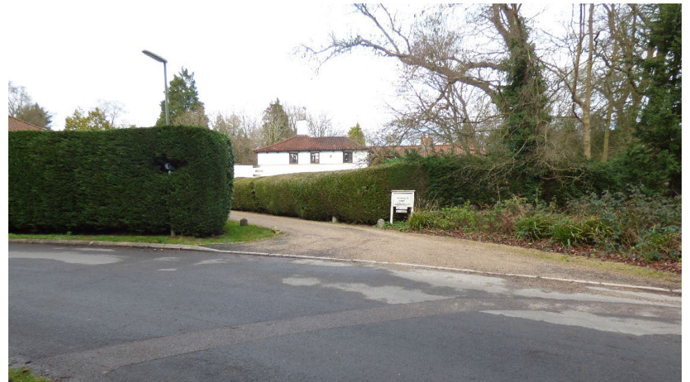
Figure 54: The listed lodge buildings on Ridgemean Road form the entrance to Ridgemean House.
